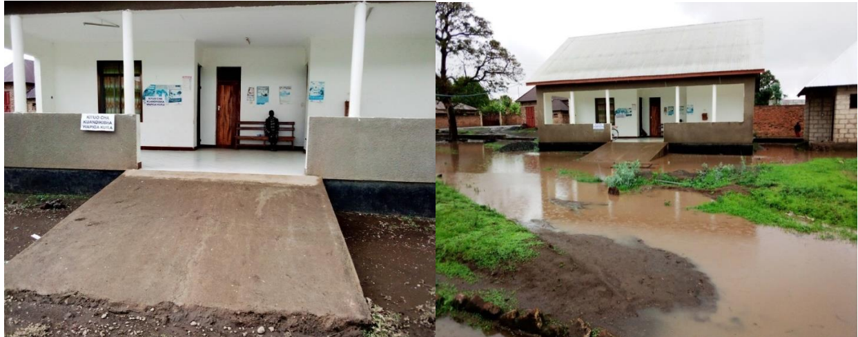
In the left photo: Itensa Dispensary registration, before it started raining and at the right photo the same center surrounded by rainwater at around five in the evening. Mbeya City Council, December 8 th , 2019.
